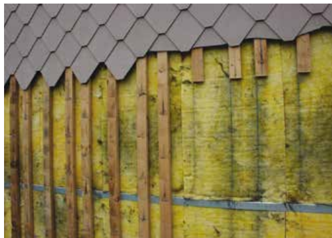
Example from a sample collection documentation: ventilated facade
